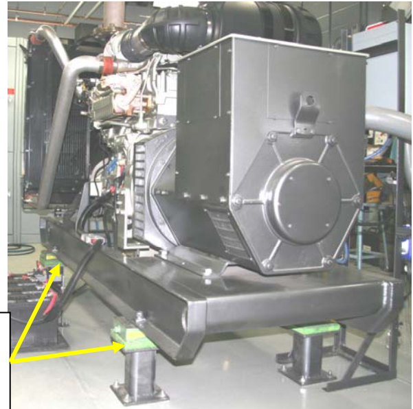
AirLoc Wedgmound® Family with Pads Wedgmounds/Damping Pads under John Deere Genset
