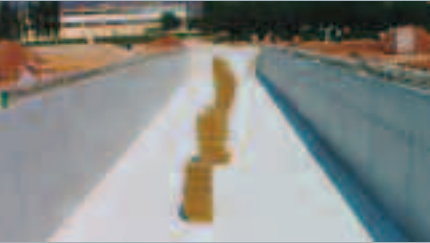
Figure 1: Foundation tank before installing the vibration isolation pads
