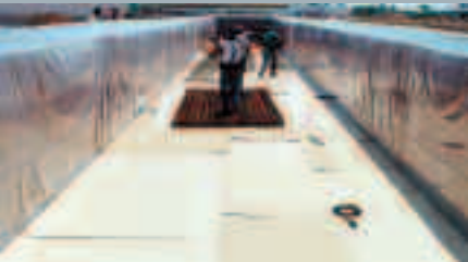
Figure 3: Block preparation for pouring the foundation
