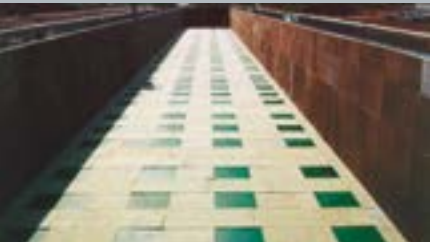
Figure 2: After installing the isolation (green)
