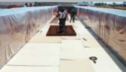
Figure 3: Block preparation for pouring the foundation
